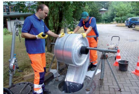
▲ Pulling in the heat exchanger
